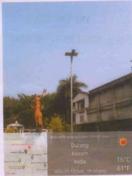
Figure: Solar lamps installed in the campus
